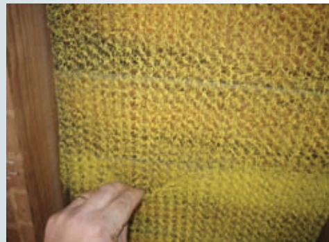
We installed a rain screen made by Homeslicker next to the siding.
